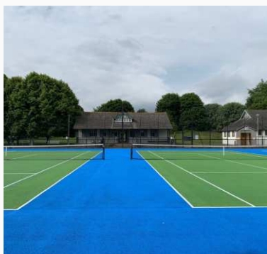
Restored Tennis Courts
